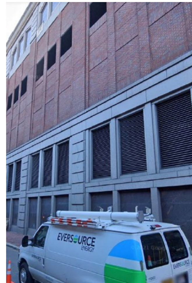
CHATHAM ST., NORTH END
