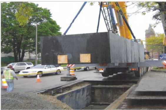
Underground vault installation
