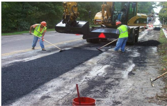
Temporary roadway restoration
