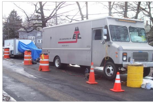
Cable splicing setup
