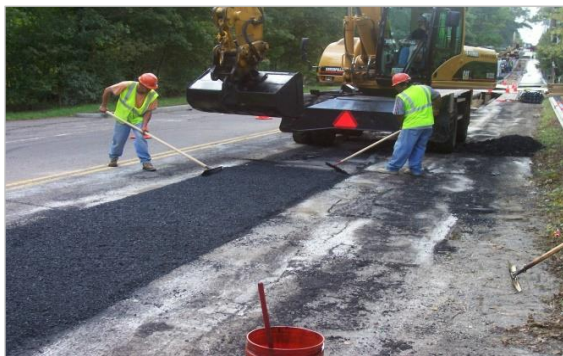
Temporary roadway restoration
