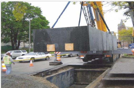
Underground vault installation
