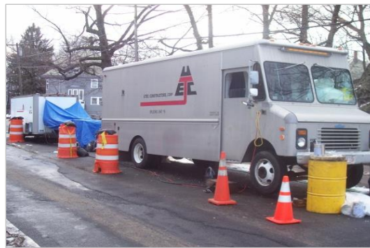
Cable splicing setup
