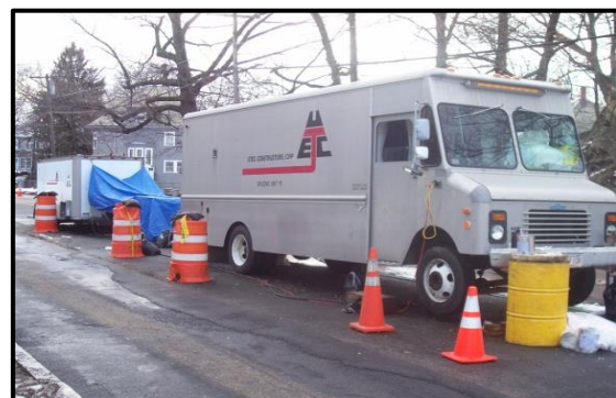
Cable splicing setup
