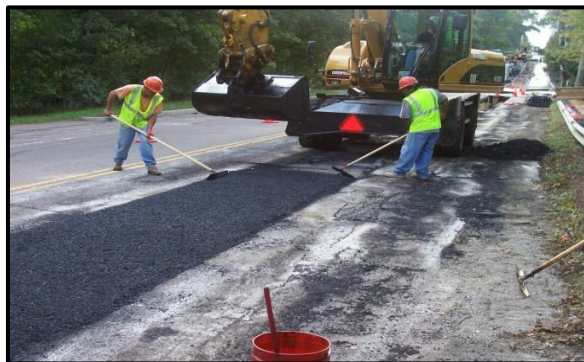
Temporary roadway restoration
