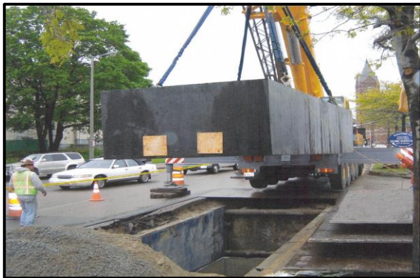
Underground vault installation
