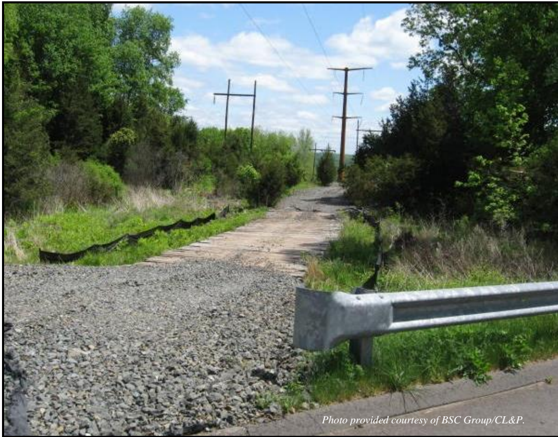
Construction entrance track pad.
