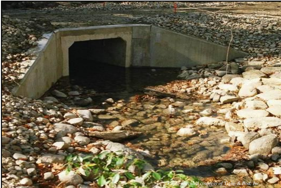
Embedded box culvert with wing walls.
