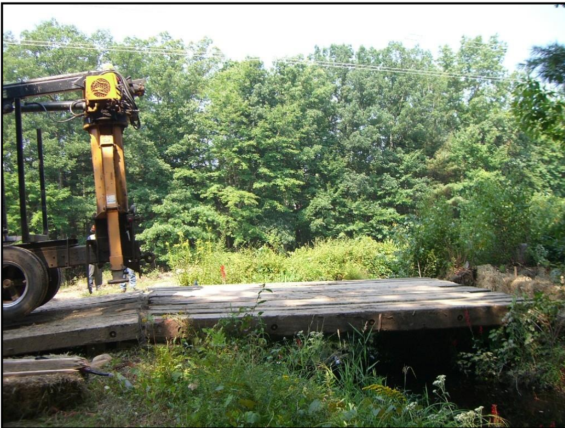
Construction mat bridge.
