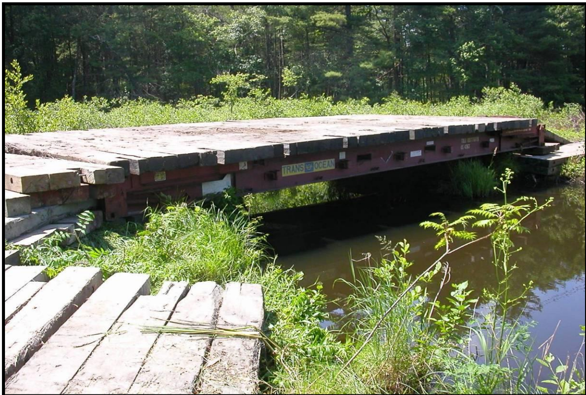
Rail car frame bridge crossing.
