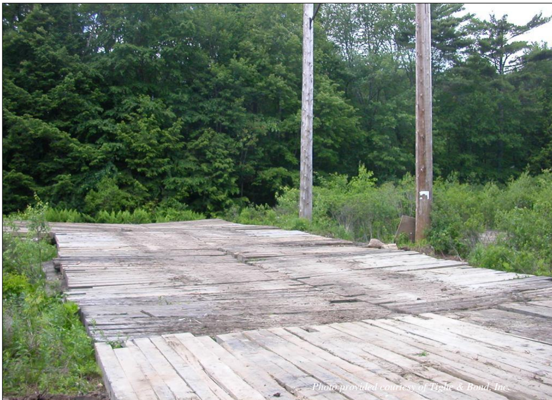
Construction mat wetland work-pad for de-energized work.
