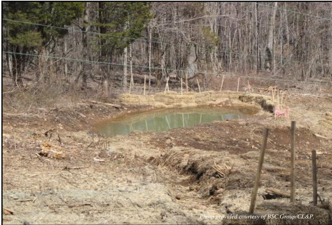
Sedimentation basin with hay bale filters.
