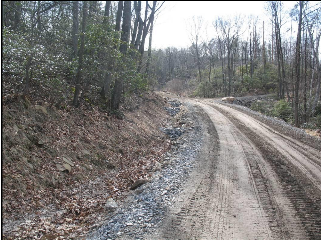
Stone check dams at construction site.
