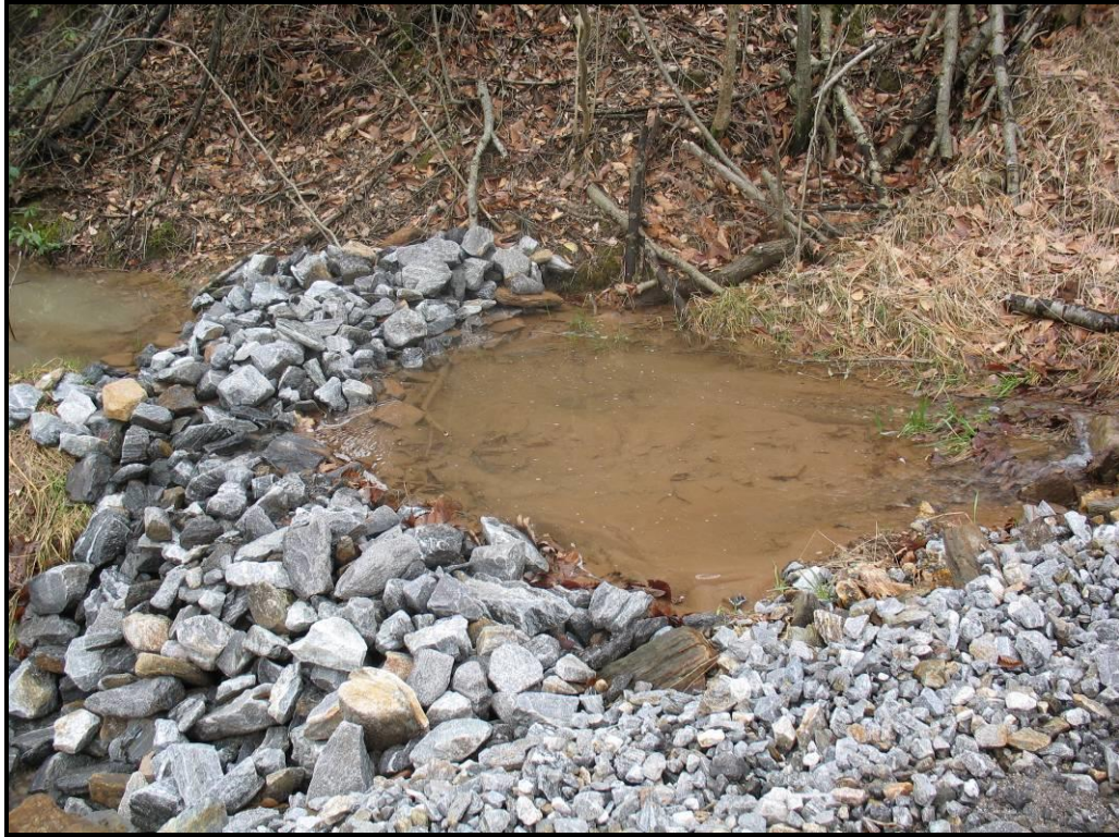
Stone check dam at construction site.
