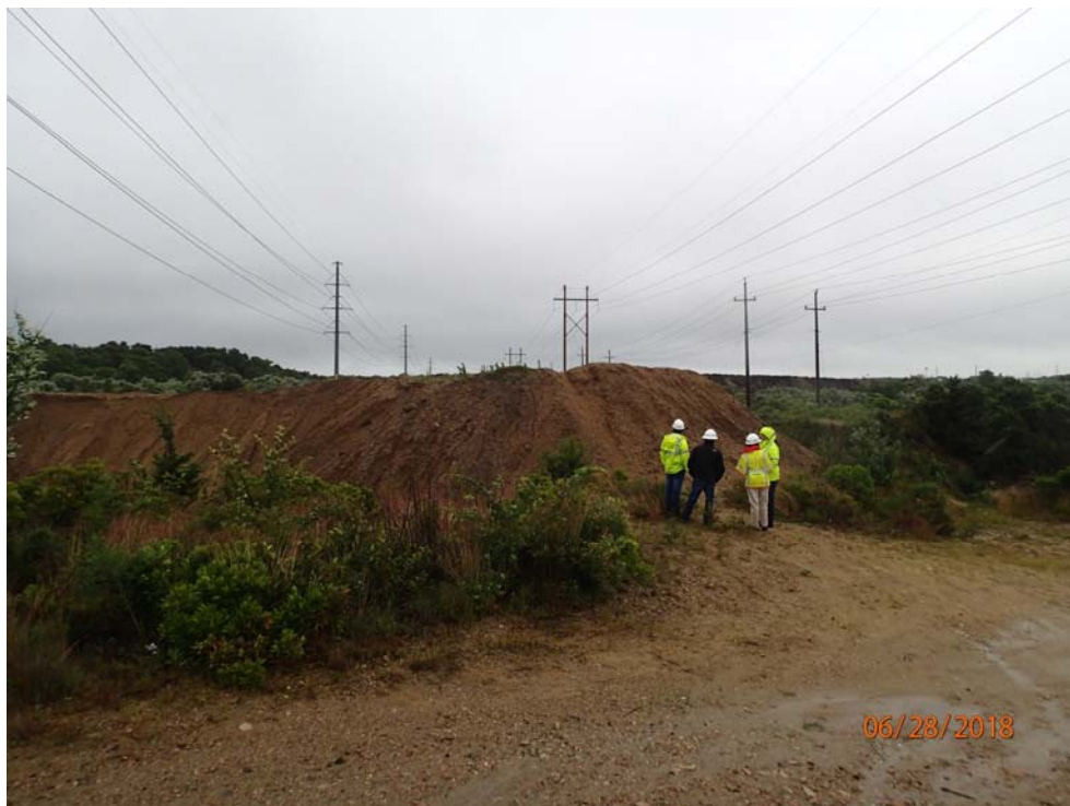
Photo 10: View looking north towards proposed structure 323.
