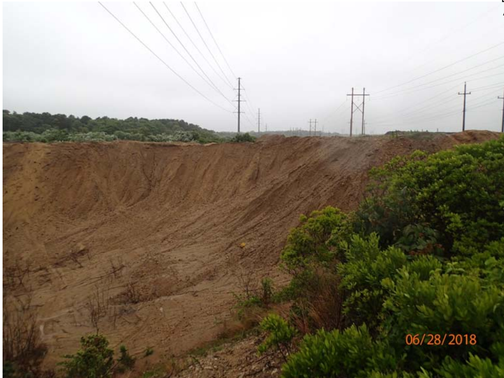
Photo 9: View looking north towards proposed structure 323.
