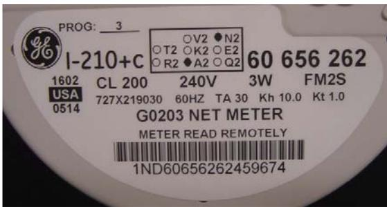
Typical nameplate for a G0203 Net Meter (kWh only)
