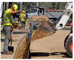
and steel pipe with new plastic pipe, which is safer, more durable, and will help strengthen the gas delivery system.
