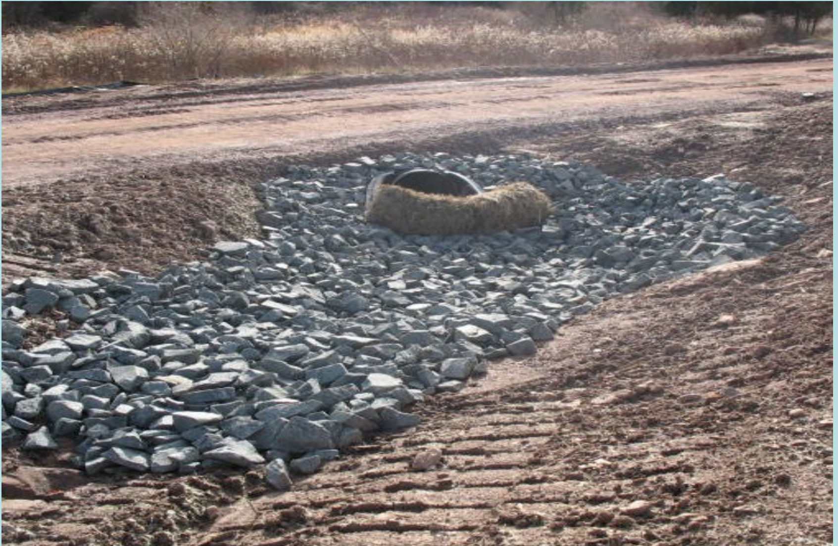
Crossing Culvert with Rip Rap and Hay Bales for Sediment Control
