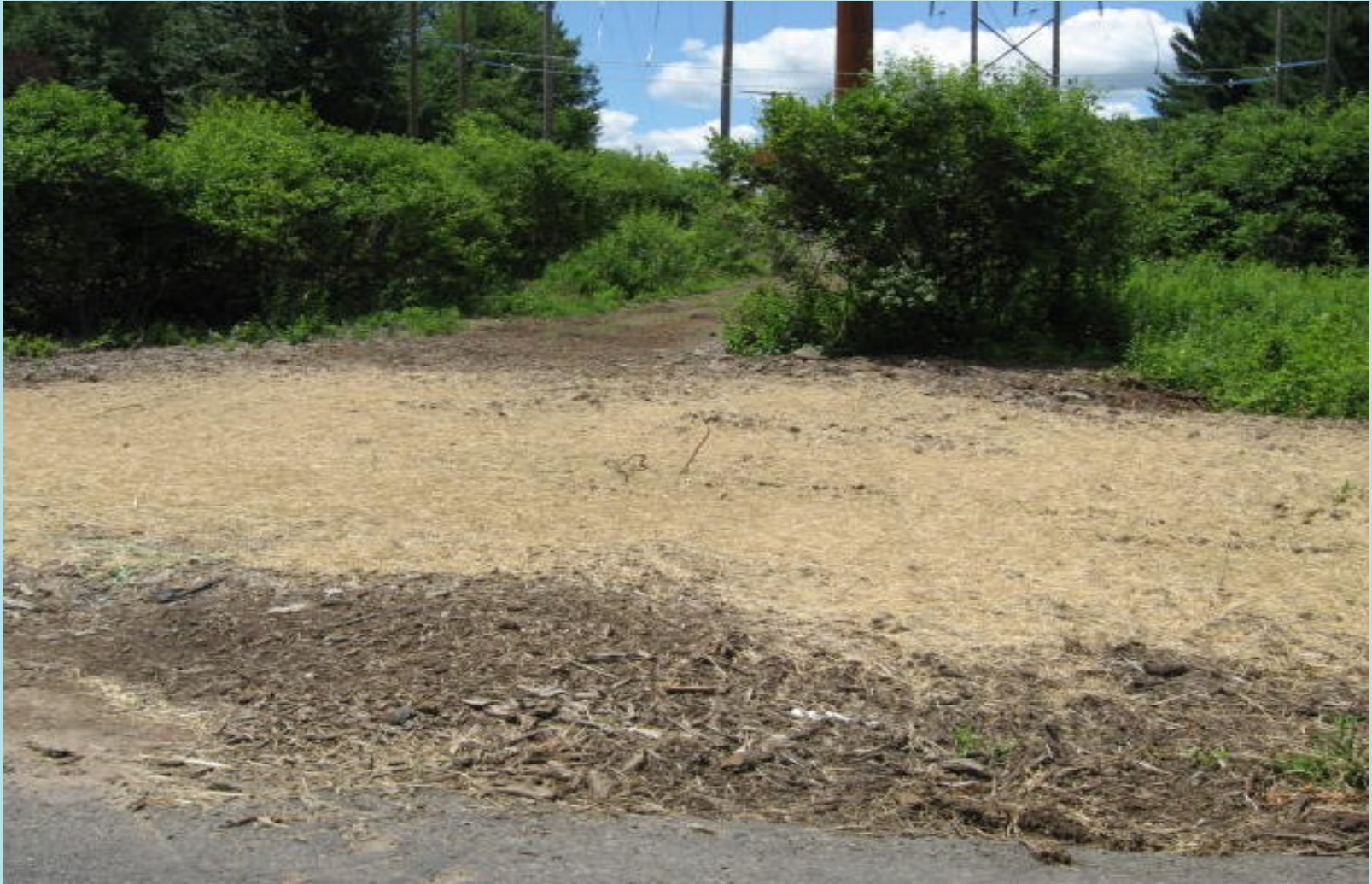
Temporary Hay/Straw Mulching for Erosion Control
