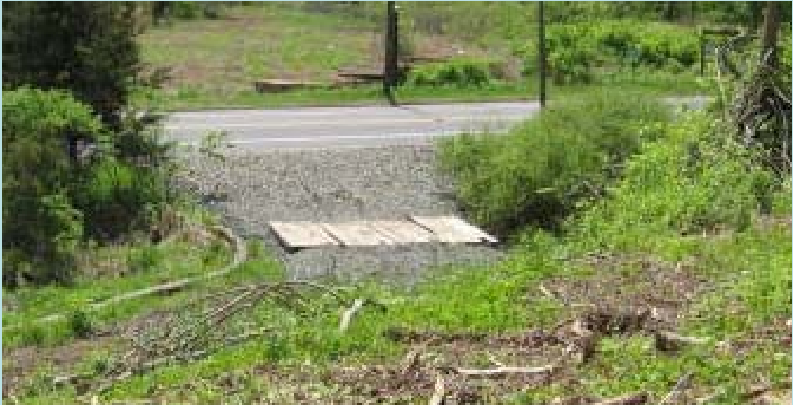
Example of Swamp Mats used as a Temporary Bridge crossing
