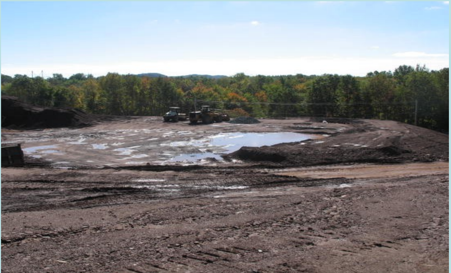
Beseck Substation Construction
