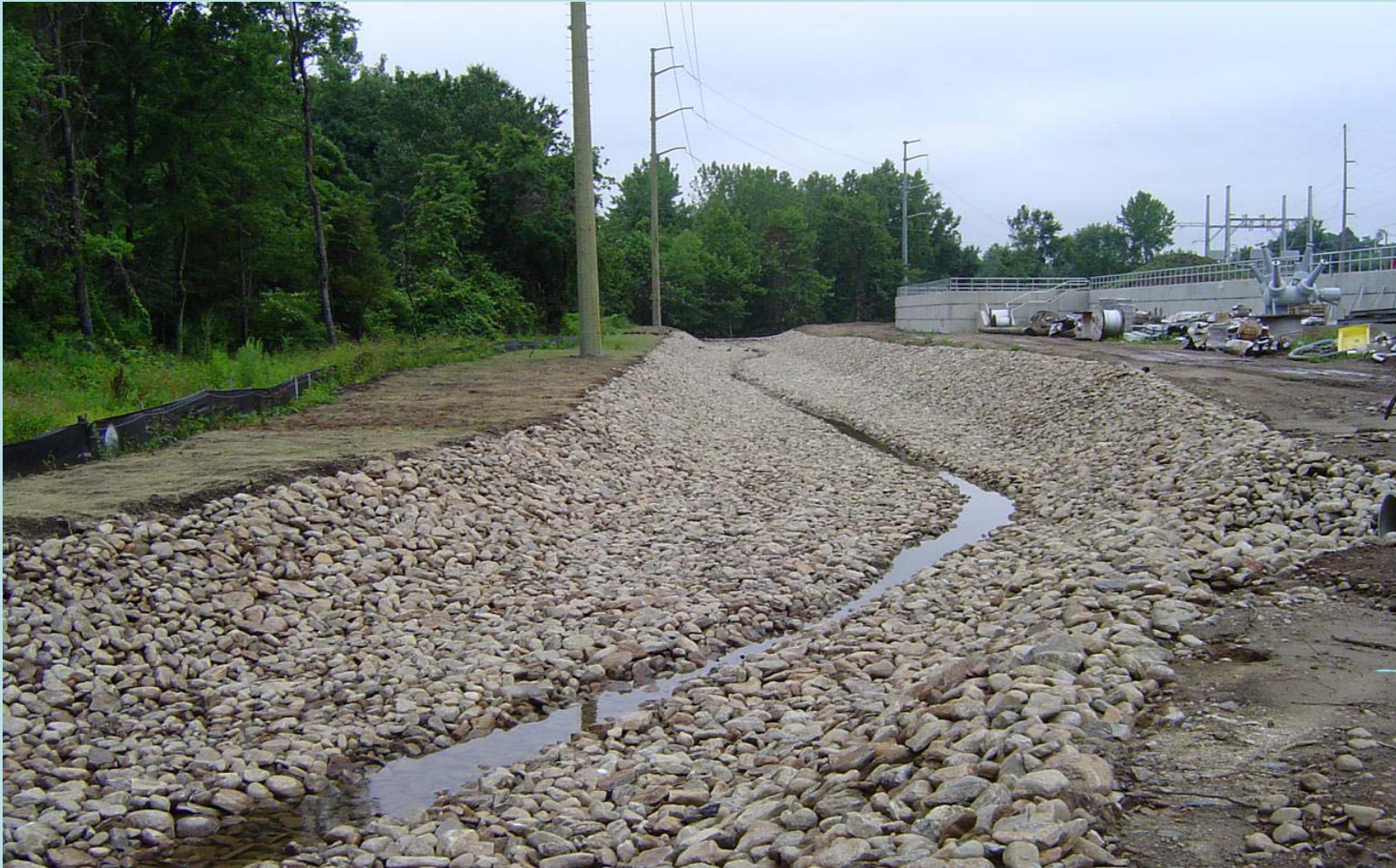
Overflow Channel for Flood Control Norwalk Substation
