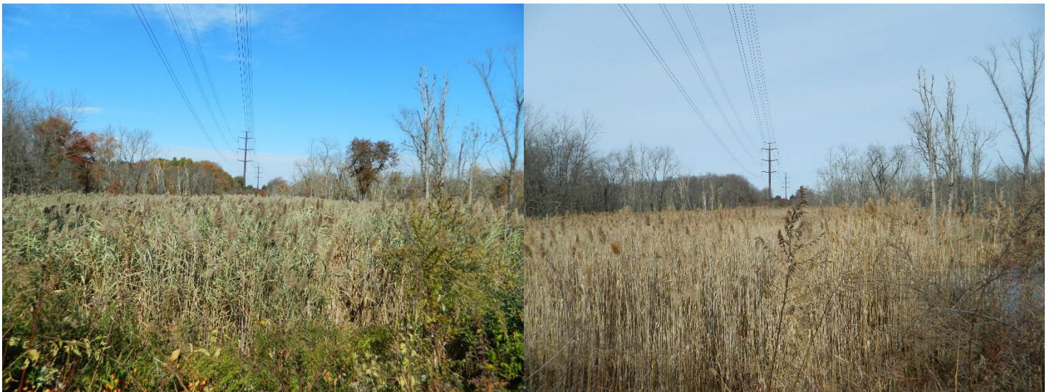
Photo 4A & B: View facing north towards the existing right-of-way as seen from Shelter Rock Road in Bethel and Danbury.
