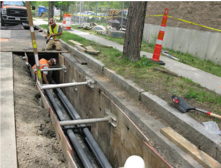
Typical trench for underground cable installation
