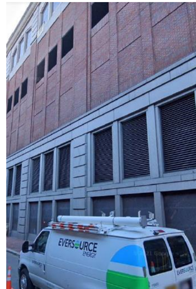
CHATHAM ST., NORTH END
